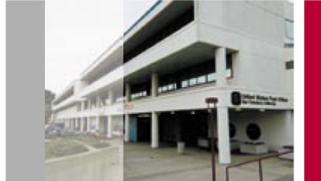
U.S. Postal Service San Francisco Processing & Distribution Center
