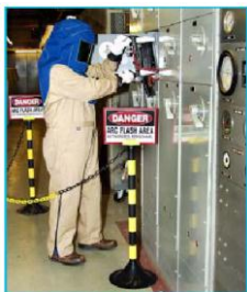
Act: Wear in protective clothing and gear as he inserts a starter socket into a Motor Control Center.
